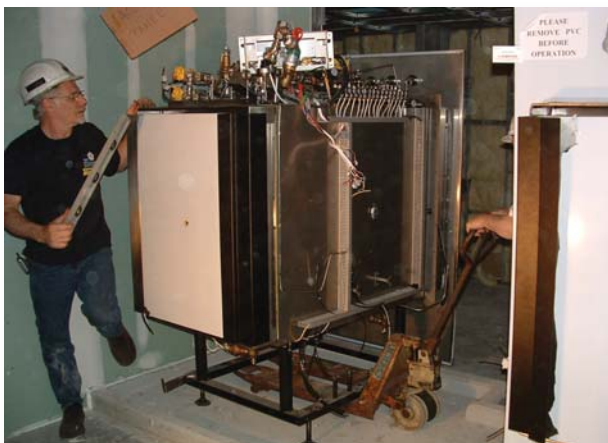
Installation of Pass-Thru Sterilizer
