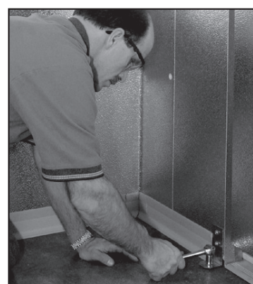
Attach slam brace with fastener provided
