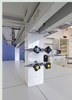
Gas needle valves in double-sided table
