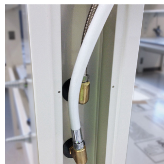
Gas needle valves in double-sided table
