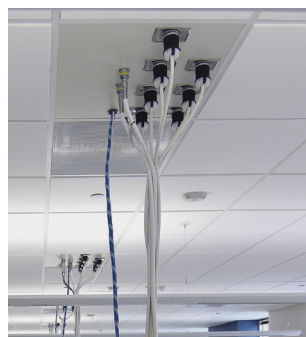
Ceiling service panels installed into ceiling grid to distribute services to table locations
