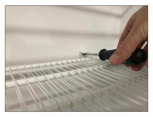
STEP 2. Installation of the Rear Retaining Channel
