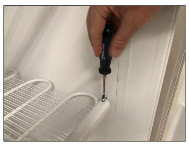
1b. Carefully loosen shelf from existing rear support brackets and remove and retain 2 screws, discard the brackets.
